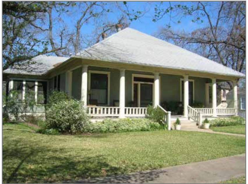
4206 Ave D, the Huston House
