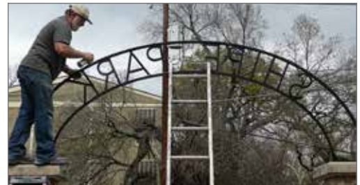
Stan installing the Shipe Park arch
