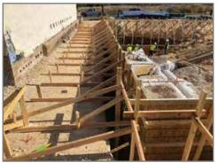
Pool Forming prior to Rebar Installation
