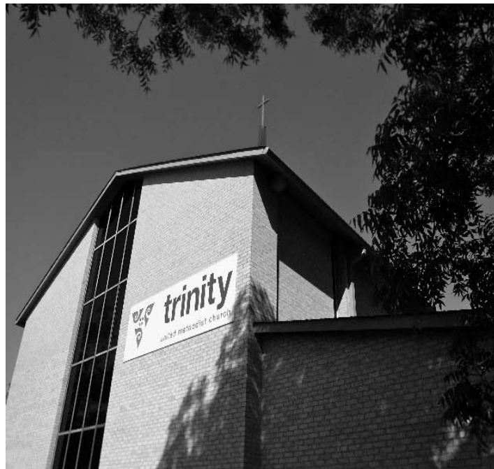
The newly arrived Trinity Methodist congregation at 40th and Speedway, has completed a beautiful renovation and retains the historic stained glass
