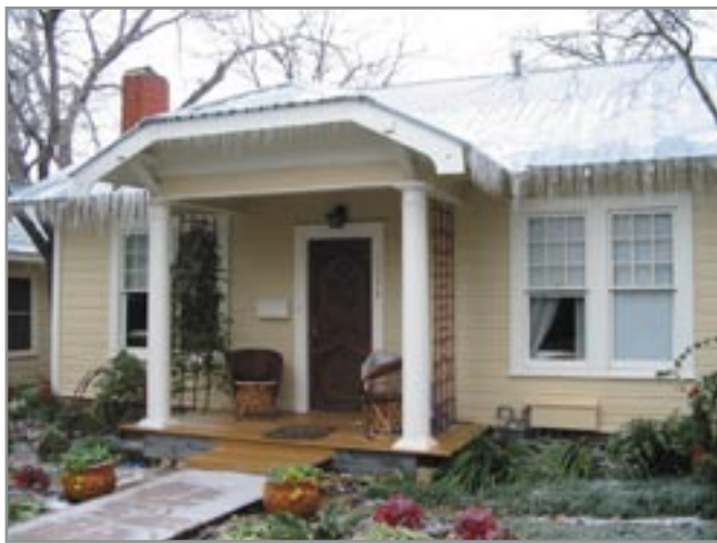
Robey House in Wintry Trim. photo by Lorre Weidlich
